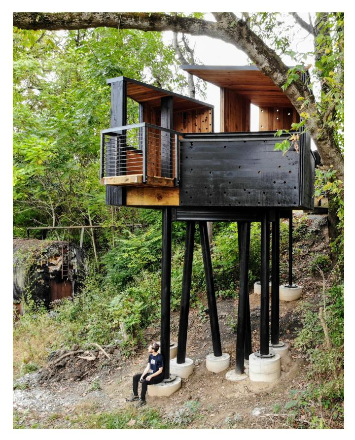
Figure 4. New River Train Observation Tower constructed with locally-sourced, custom-developed hardwood CLT.
