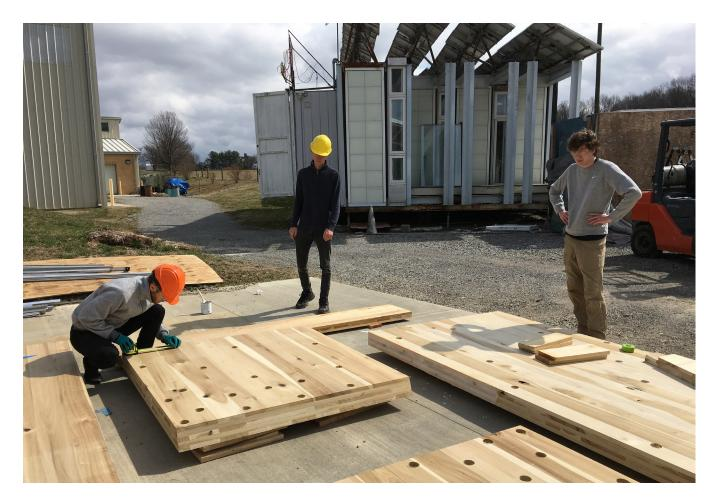
Figure 3. Custom-developed hardwood CLT from local forests before assembly.
